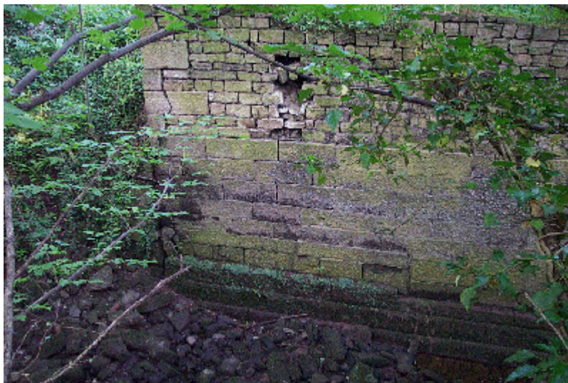
Roman mill in Northumberland with later additions
